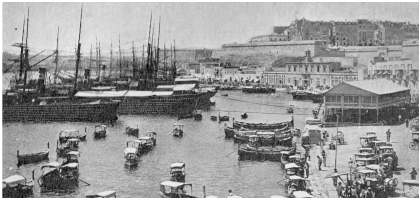
Figure 8. Scenes of Transportation Infrastructure in the 1900s
