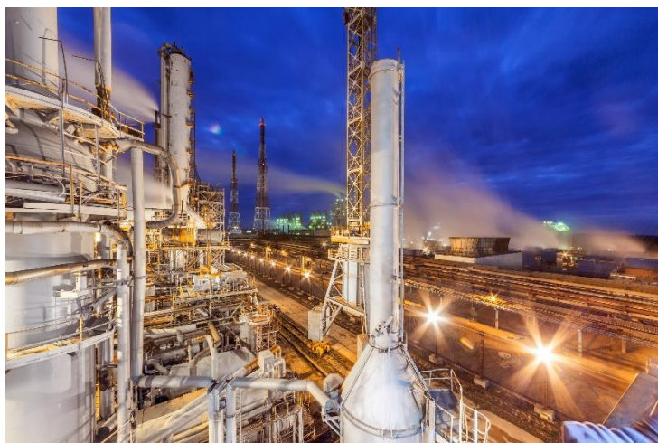
Figure 4-2 KIMA 1200 tpd ammonia plant in Aswan Governorate, Egypt
